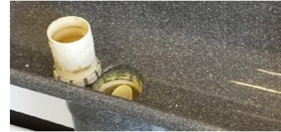
Remove stainless steel waste cover (step 2)
